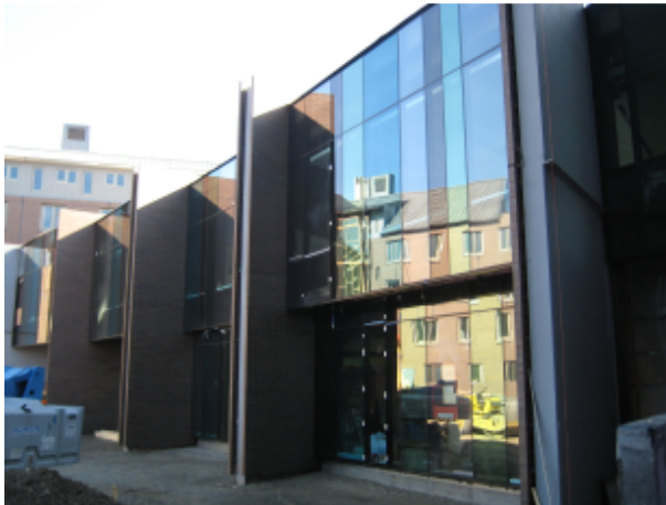
Dining Pavilion – Brick clad piers with curtain wall façade.
